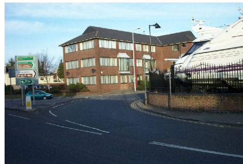
Hamworthy Bridge approach (from south)
