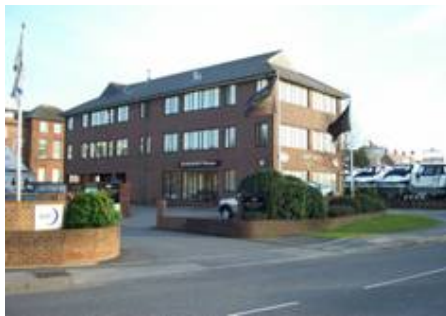
West Quay Road (from north) Car park entrance (shared with Deverill)
